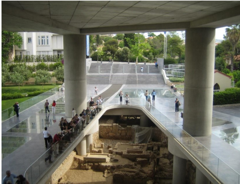
Figure 6. A portion of the excavation open for viewing under the canopy of the main entrance of the Acropolis Museum
